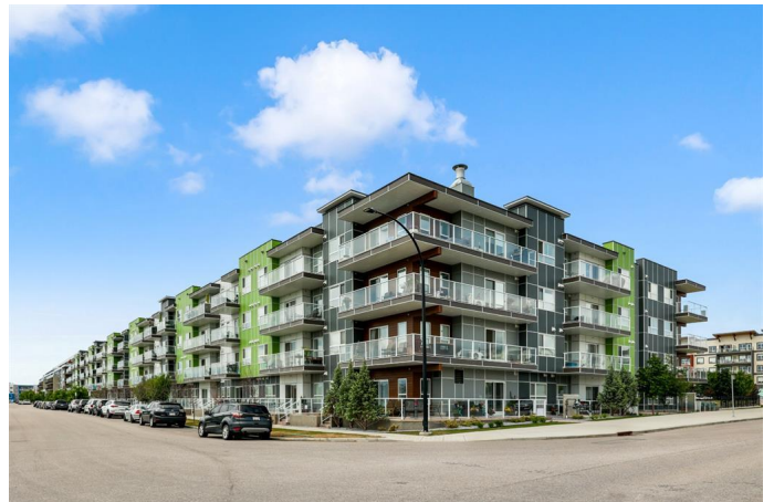
#214, 20 SETON PARK SE REC-MEASUREMENT STANDARD - CALGARY AB MAIN LEVEL (AG) - 822.28 Sq Ft / 76.39 m 2 TOTAL ABOVE GRADE RMS SIZE - 822.28 Sq Ft / 76.39 m 2
